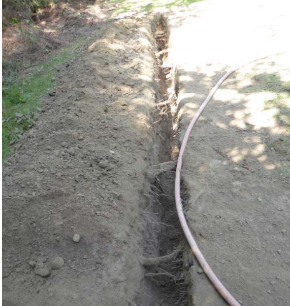
Photo 2. View looking to the north along the east trench. This view shows the low density of structural roots encountered.
