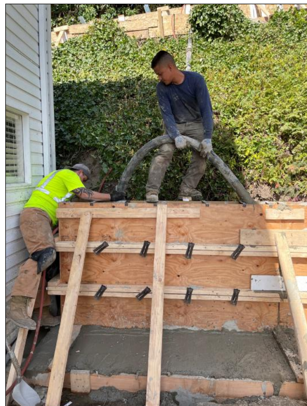
① SMALL RETAINING WALL
