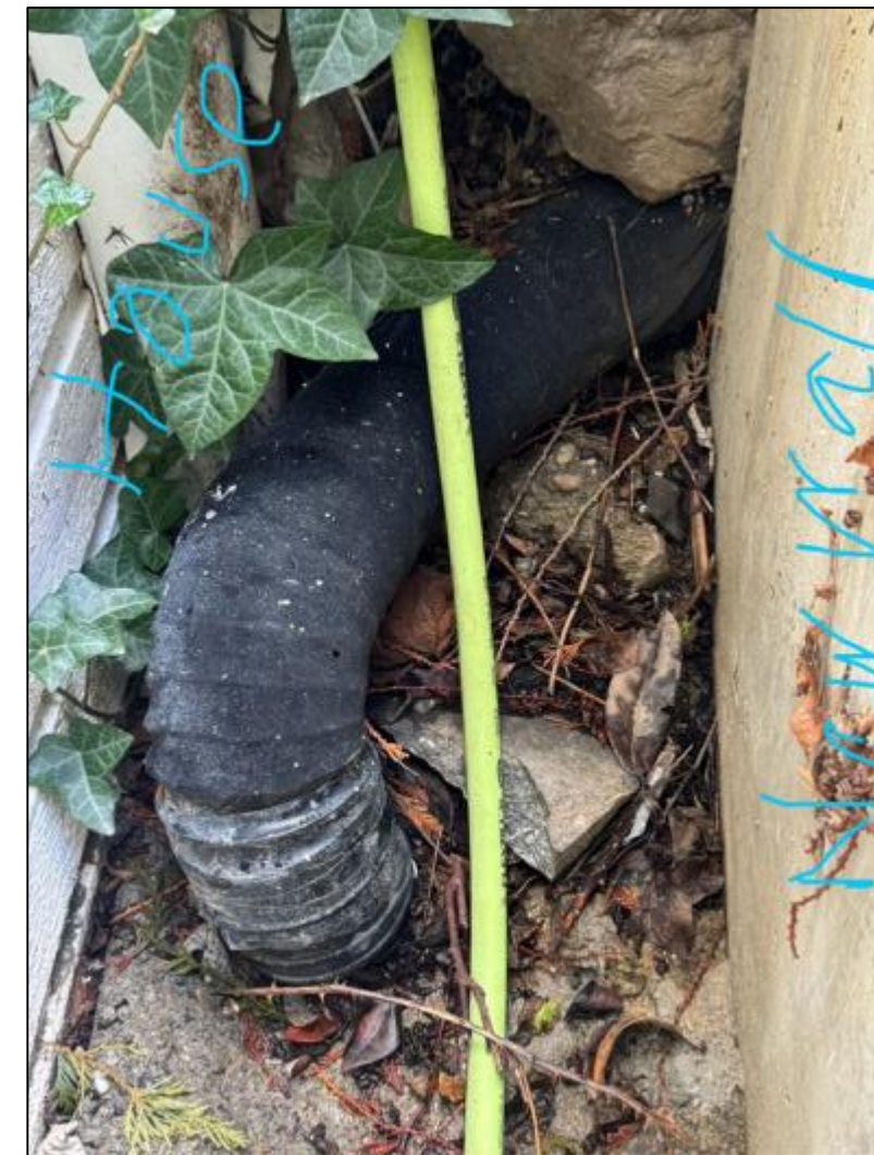
① DRAIN PIPE @ RETAINING WALL
