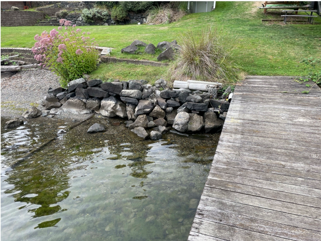
Photo 4 - Existing shoreline south of the dock.
