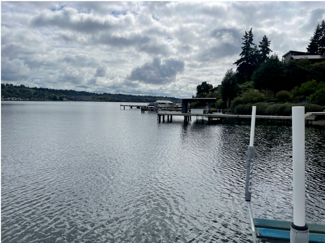
Photo 6 - Existing conditions south of the site.
