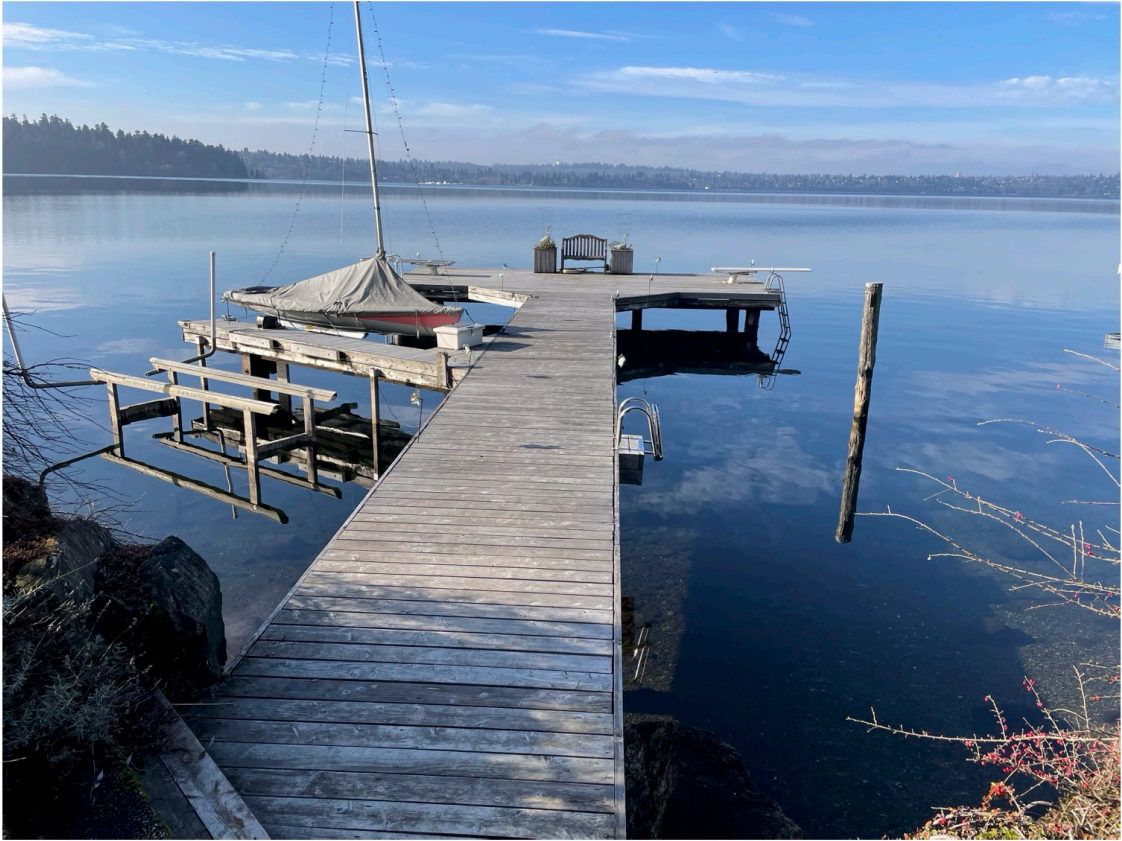
Photo 1 - Existing dock looking waterward.
