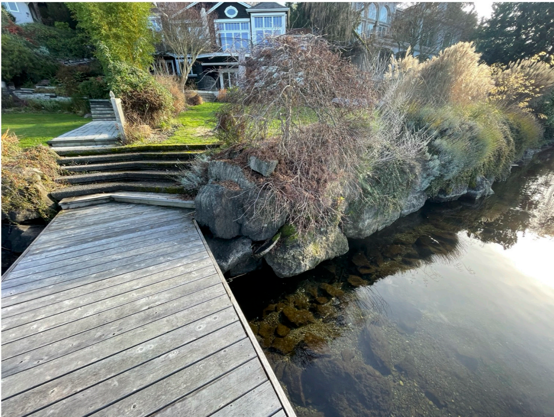
Photo 4 - Existing dock looking south.
