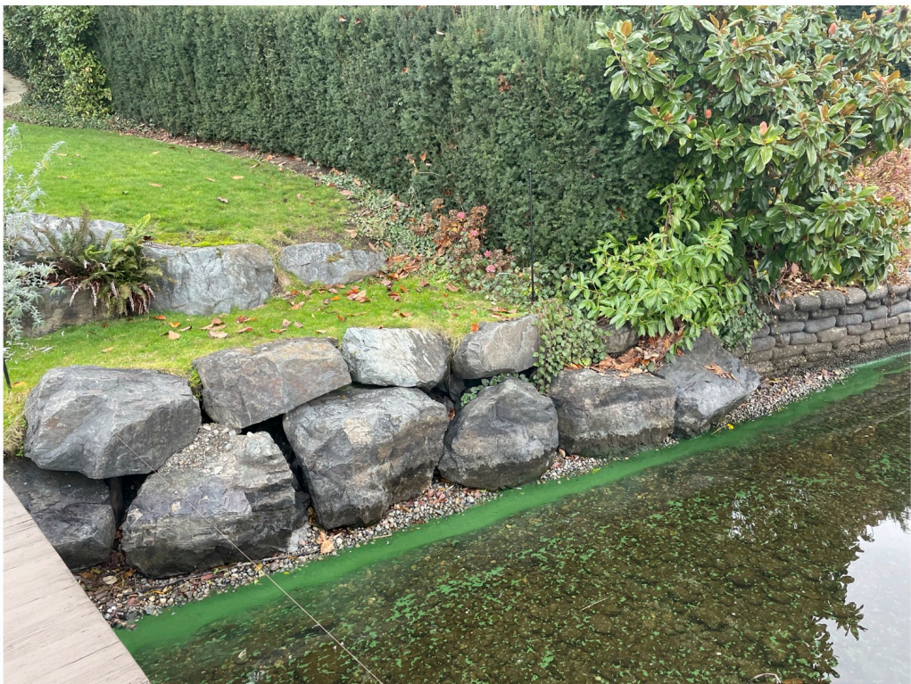
Photo 4 - Existing shoreline looking south.
