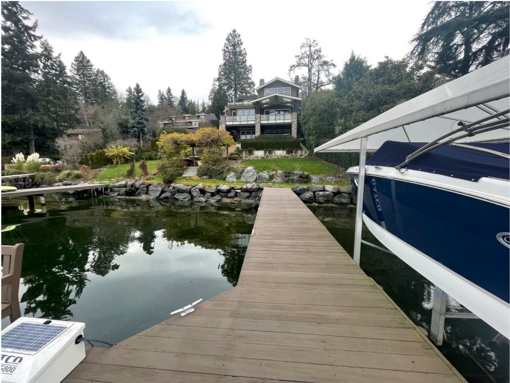
Photo 2 - Existing dock looking landward.
