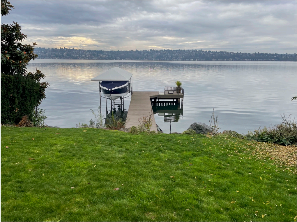
Photo 1 - Existing dock looking waterward.
