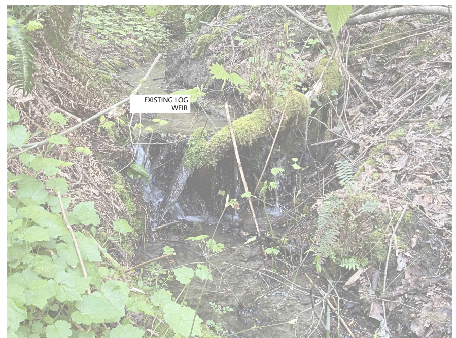
EXAMPLE PHOTO (STA 5+45)
