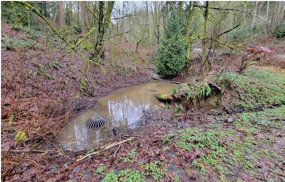
Photo 1.1 Upstream view of East Mercer Way crossing and upstream sediment pond.
