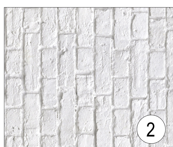
2 PAINTED EXISTING BRICK
