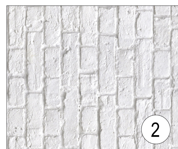
PAINTED EXISTING BRICK
