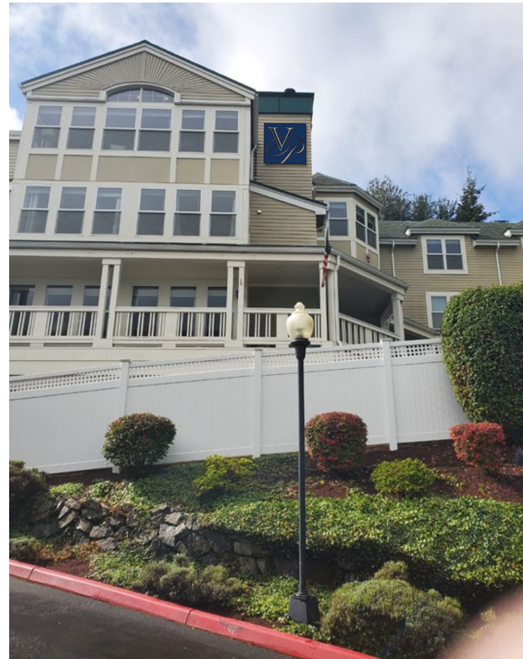
Proposed Install Location - Details Pending Survey
