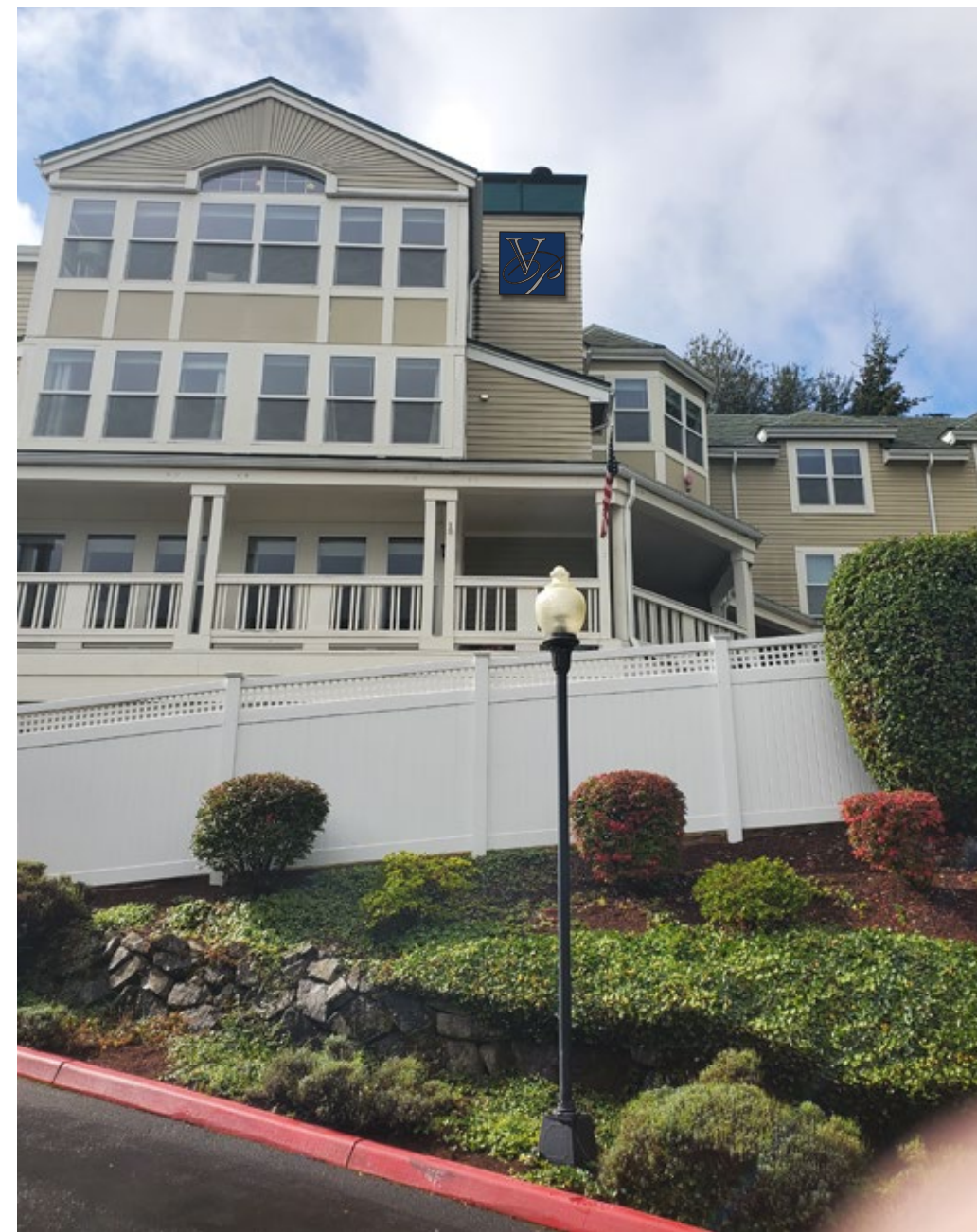
Proposed Install Location - Details Pending Survey
