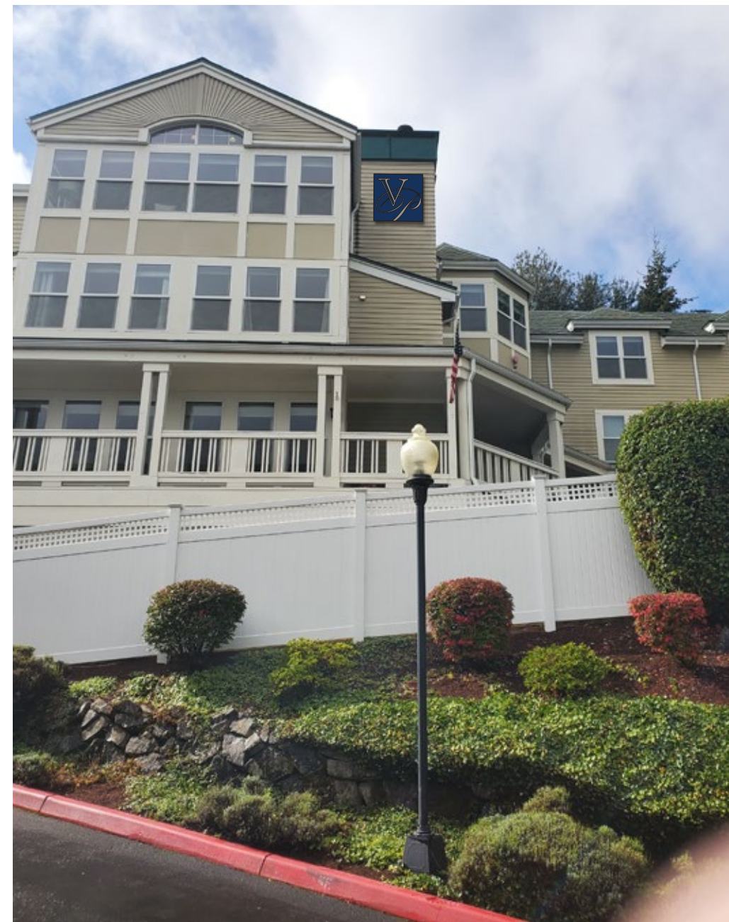
Proposed Install Location - Details Pending Survey
