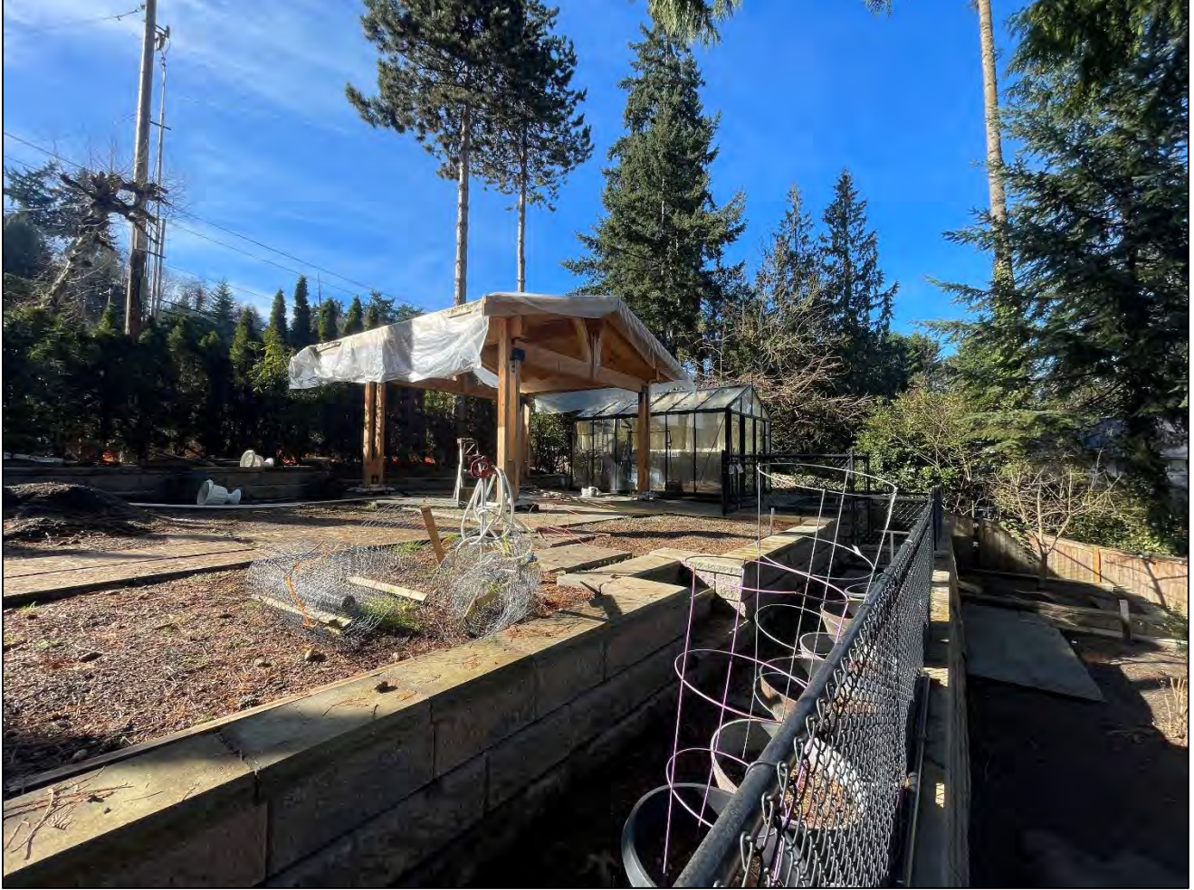
Photo 3. Looking southwest toward recent site work.
