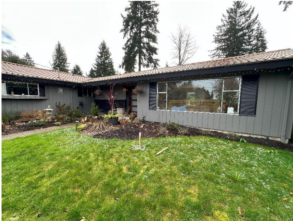
Plate 2. View of the proposed north side improvement area, looking southeast.
