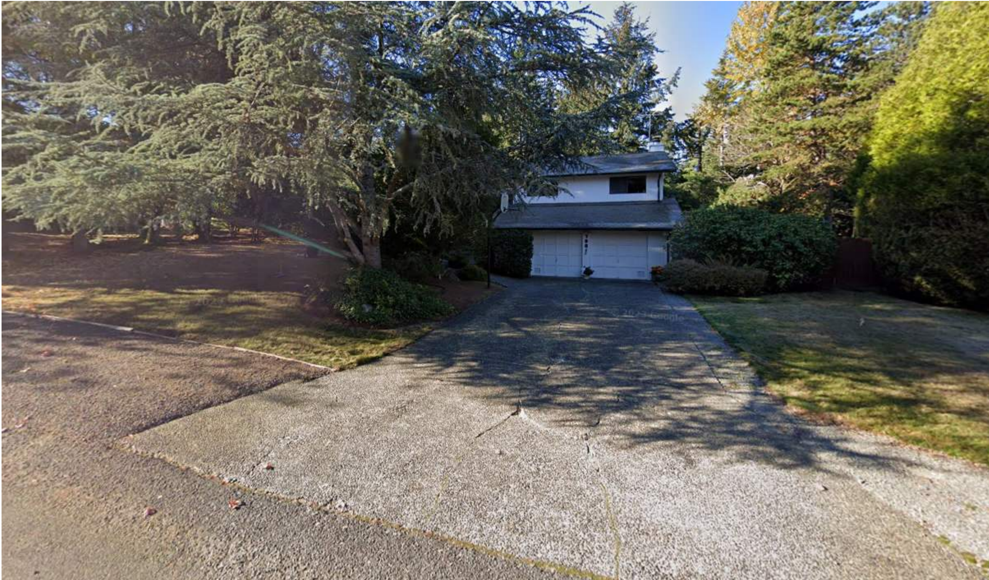
1 MAIN HOME - FACING EAST
